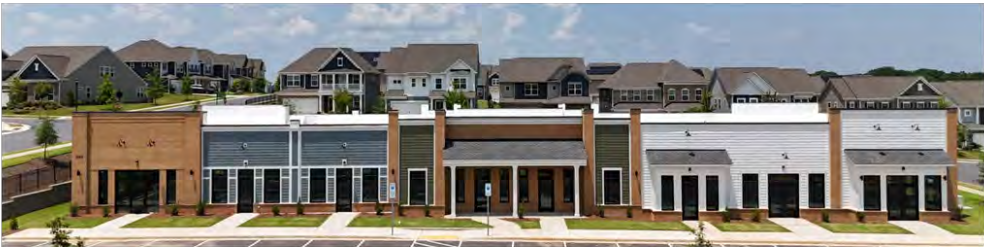
Source: Kuester Commercial, Windhaven Village
